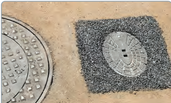
Vault with Remote Antenna Box.
