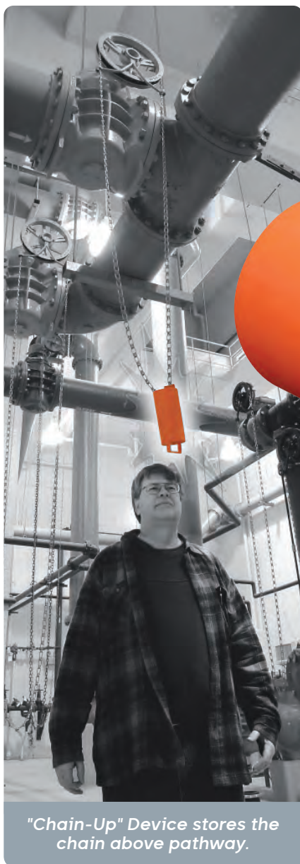
Chain from overhead Chainwheel shown in pathway.
