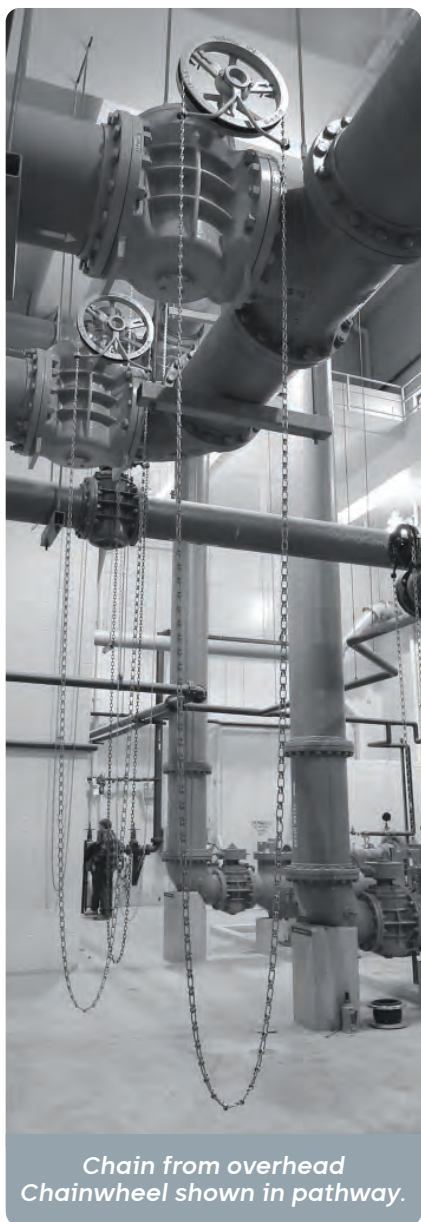
"Chain-Up" Device stores the chain above pathway.
