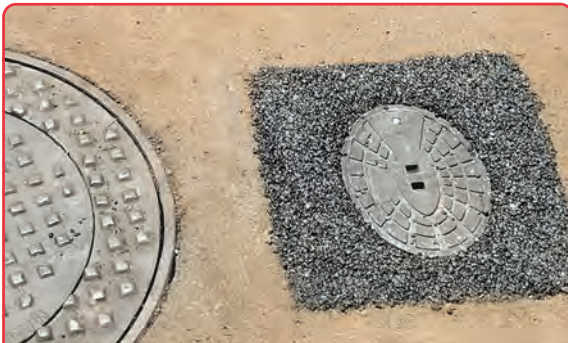
VAULT WITH REMOTE ANTENNA BOX.
