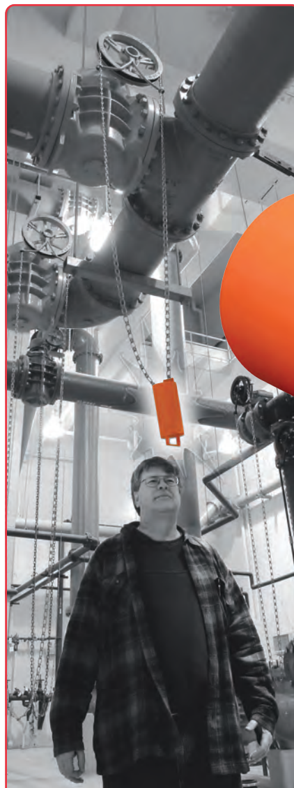
"CHAIN-UP" DEVICE STORES THE CHAIN ABOVE PATHWAY.
