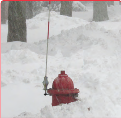
HYDRANT MARKERS HELP FIND HYDRANTS WHEN THEY ARE NEEDED MOST.
