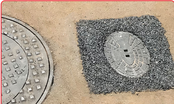
VAULT WITH REMOTE ANTENNA BOX.
