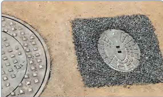
Vault with Remote Antenna Box.
