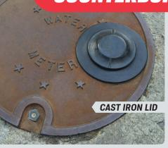
Drilling holes in existing cast iron lids may save money in the short run. However, most iron lids do not have the thickness for a counterbore. If lids are simply drilled without a counterbore, the result is a trip hazard. Drilling iron lids in the field frequently results in cracks in the lid.
